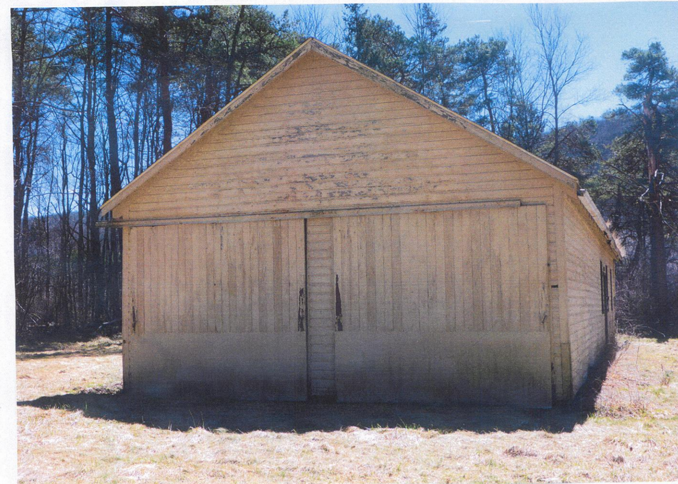
PICTURE OF BUILDING (NORTH SIDE)
