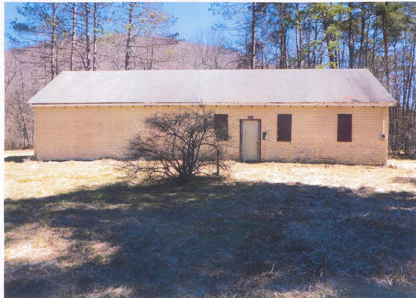
PICTURE OF BUILDING (WEST SIDE)
